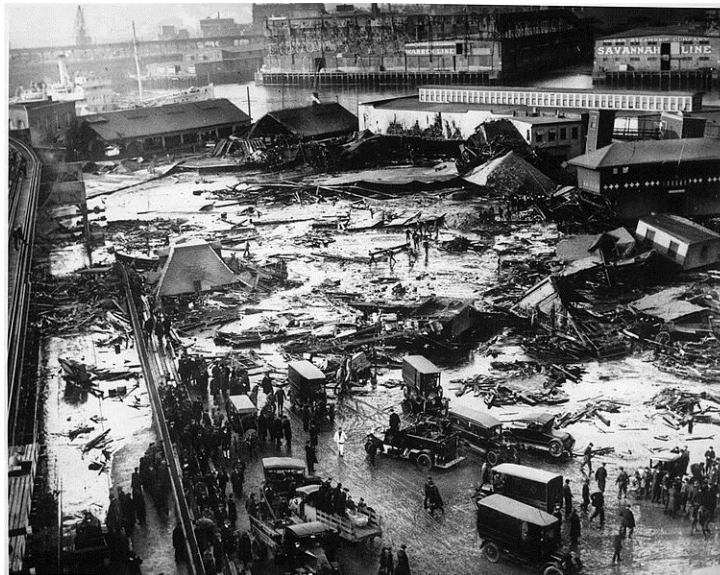
Figure 1. Aftermath of molasses tank failure
